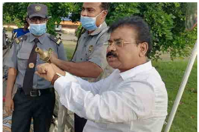
Mr. Sekhar Dey demonstrating how hold branch pipe of hydrant point.
